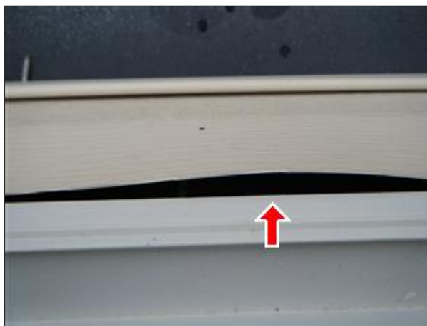
2.0 Picture 1 Looking down from window
